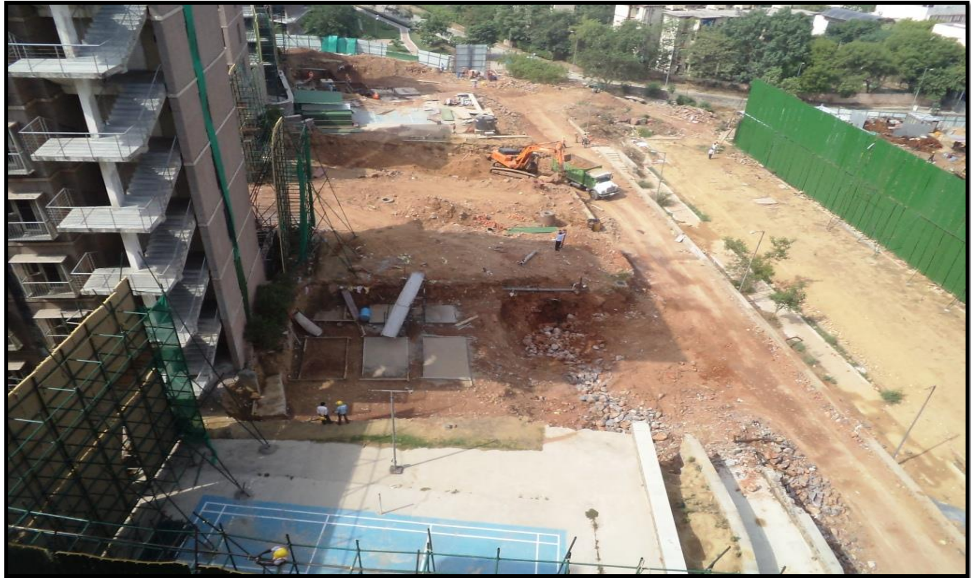
Extension Hostel Blocks G1, G2 & B1
